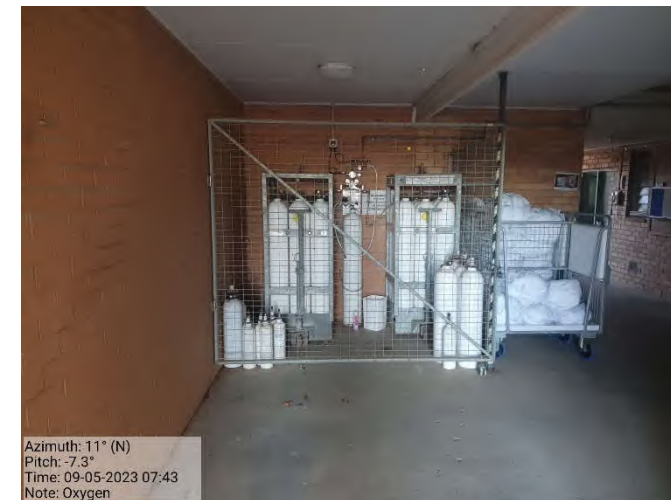
Photograph 10: Oxygen gas storage
